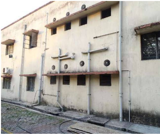
Rain Water Harvesting Pipelines & recharge Pits
